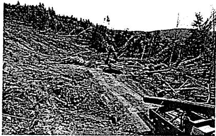
Mid August Repair work
